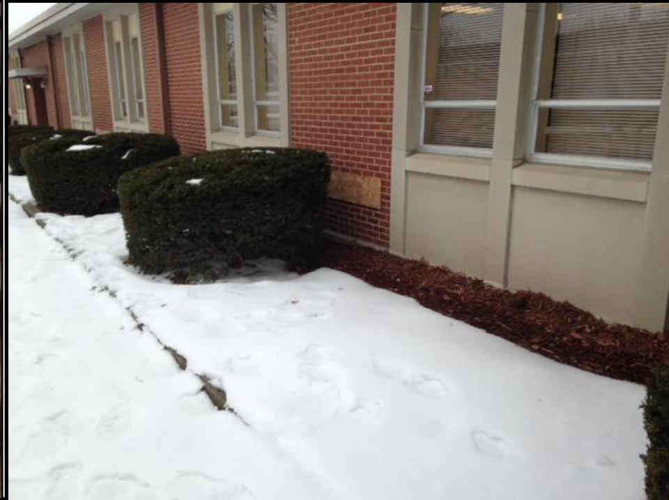
Boards to Keep Cold Air Out
